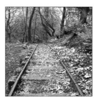
Remains of the narrow gauge railway running from Bulkeley Hill to Peckforton Water Works. Wagons were attached to cables and hauled up the incline by a winding engine.
